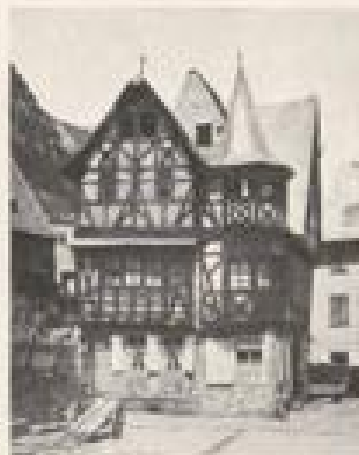
HAUS IN BACHARACH
