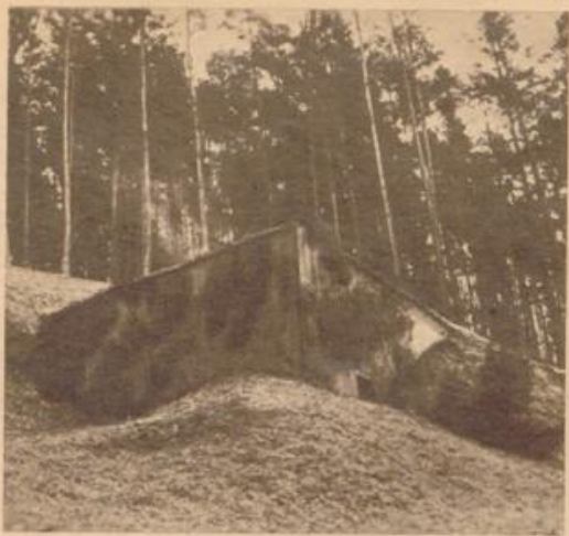
Bunker am Westwall
